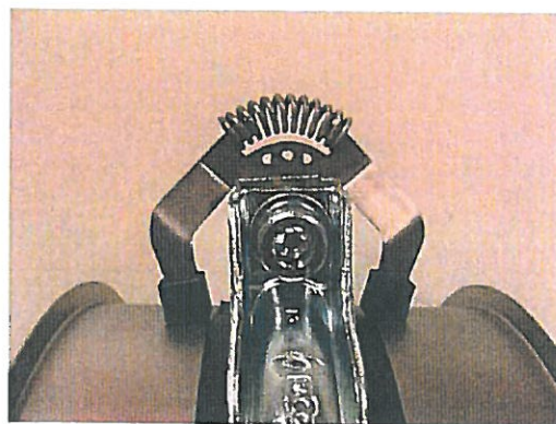
Figure 2: Earthing jumper fixed to pipe sections
